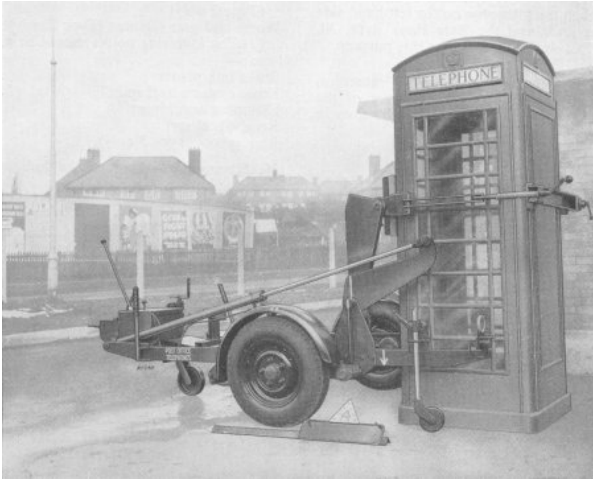
FIG. 8. LOADING A KIOSK ON TO A TRAILER
